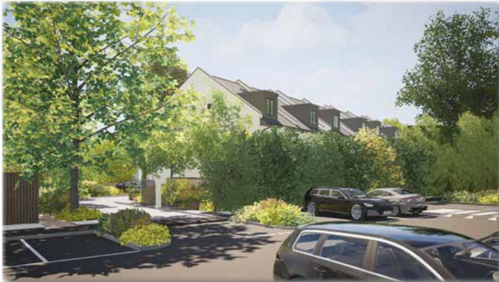
Units from car park
